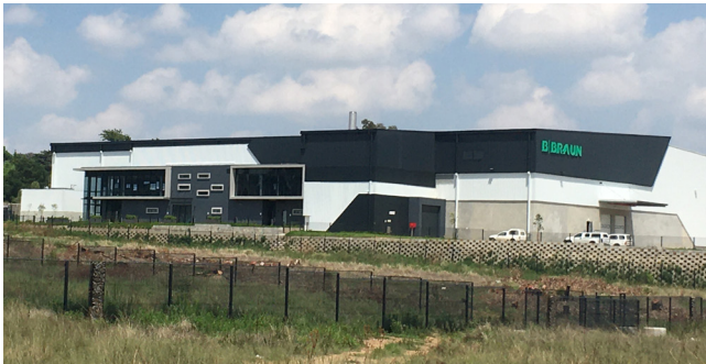
B. Braun's new liquid pharmaceuticals factory in Johannesburg, completed in 2021
